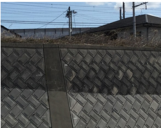
(2) The light-colored parts of this wall have been decontaminated, but the places that are too high to reach or cannot be reached with a scrubber have been left untouched. (Fukushima City, March 2017).
