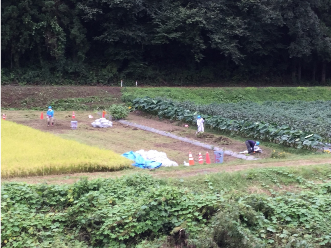
(3) Decontamination workers scraping the soil next to vegetable and rice crops. The vegetables and rice will be sold. The decontaminated soil will be added to a nearby pile of black bags and covered with a plastic sheet (Fukushima City, September, 2016).
