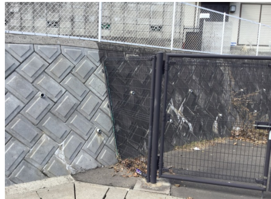
(2) The light-colored parts of this wall have been decontaminated, but the places that are too high to reach or cannot be reached with a scrubber have been left untouched. (Fukushima City, March 2017).
