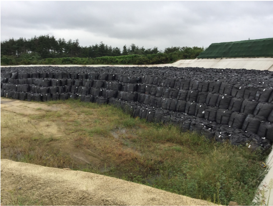
(1) This temporary storage area is located behind the Fukushima University campus in Fukushima City. Each black bag weighs one ton. When I took this photo in September 2016, it was still under construction and it presumably it will be filled and covered over the top.
